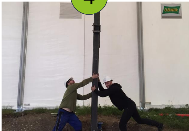
3D Printer monteres on site
